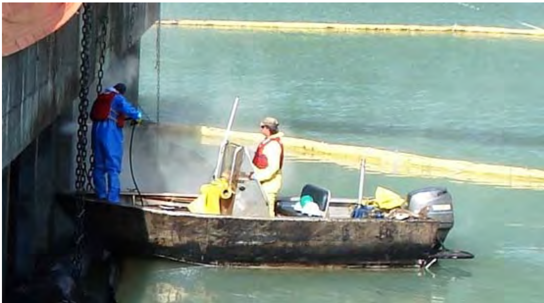
Pressure washing wharf pilings.
